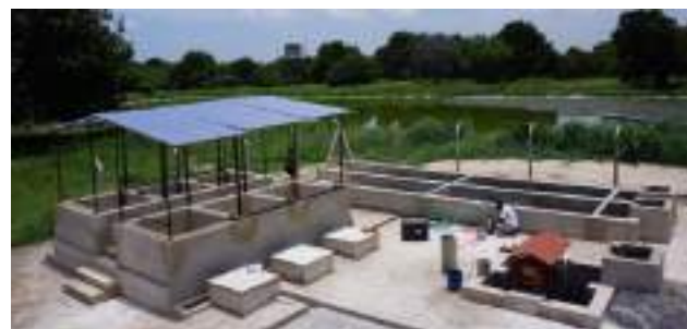
Figure 1: Dewatering facility located at University of Dar es salaam
