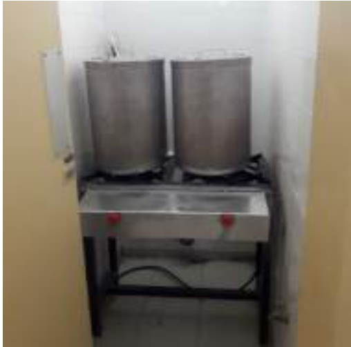
Plate 1: Biogas stove for boiling water at Mwananyamala hospital
